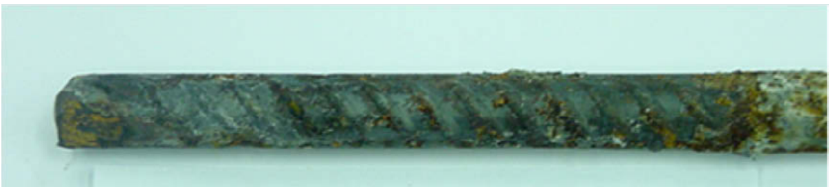
Fig. 1. Steel bar extracted from the concrete specimen contaminated with 2% chloride [17].
