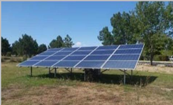
5 Kwh Solar PV Energy System Connected to Campus Electrical Grid (Dumlupınar University, Turkey)
