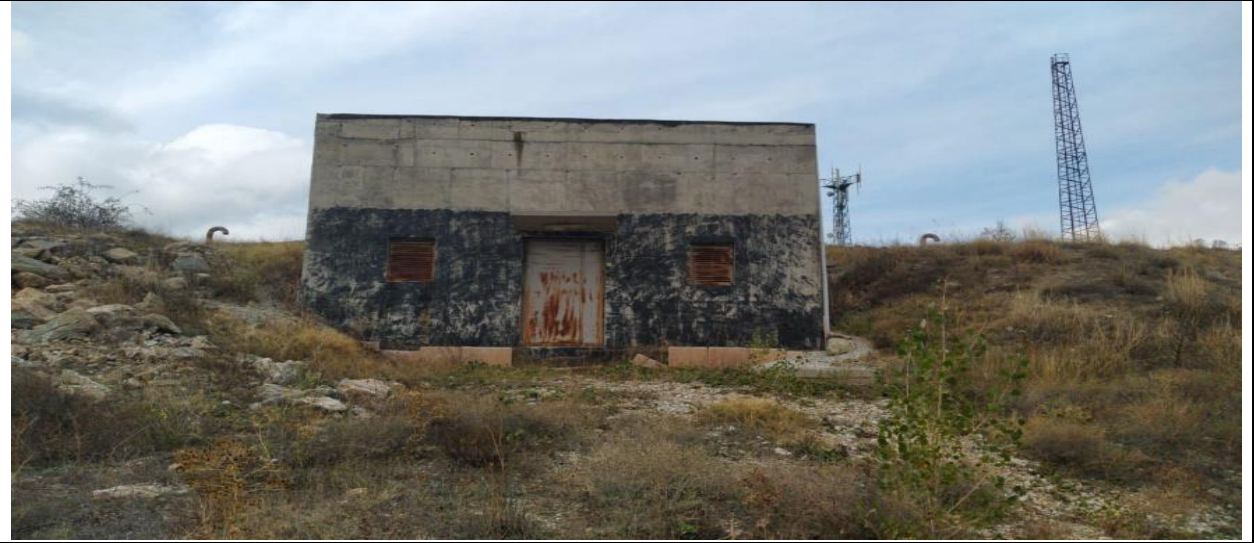
Picture A- University water reservoir (Kütahya Dumlupınar University, Kütahya)
