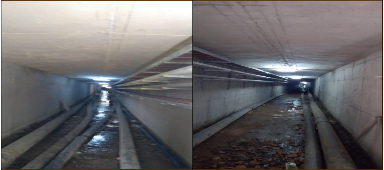
Hot water channels leading to Physiotherapy -Rehabilitation Hospital and Olympic Swimming Pool (Kütahya Dumlupınar University, Turkey)
