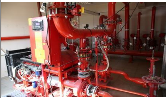
Fire Extinguishing System
