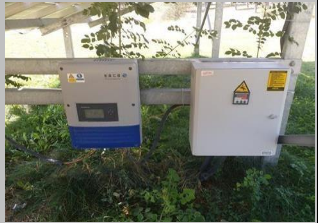
5Kwh Solar PV energy system connected to campus electrical grid. (Dumlupınar University, Turkey)
