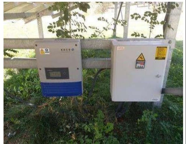
5Kwh Solar PV energy system connected to campus electrical grid. (Kütahya Dumlupınar University, Turkey)
