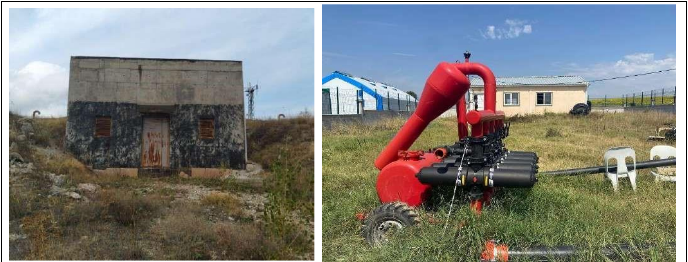
Picture A- University water reservoir (Kütahya Dumlupınar University, Kütahya)
