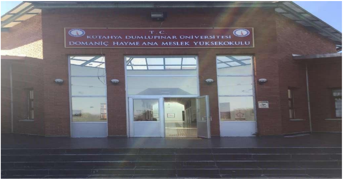
Areas created for natural lighting and heat (Kütahya Dumlupınar University)
