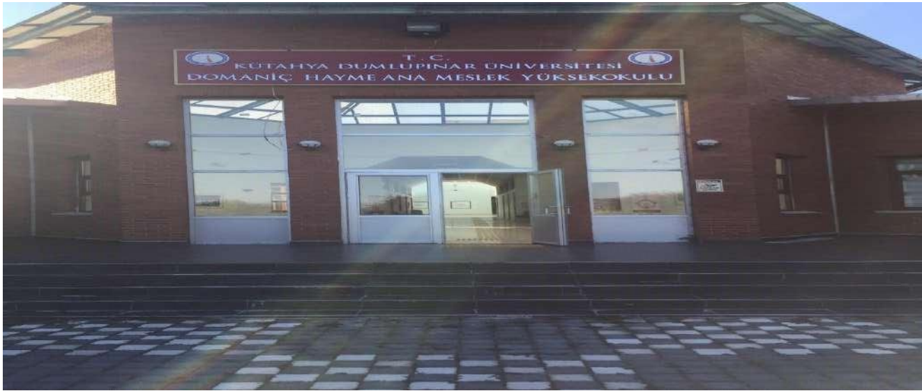
Areas created for natural lighting and heat (Kütahya Dumlupınar University)
