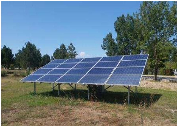
5Kwh Solar PV energy system connected to campus electrical grid. (Kütahya Dumlupınar University, Turkey)
