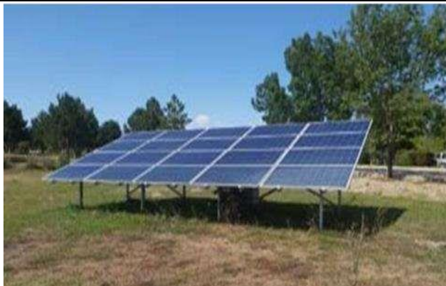
2.5 Kwh Solar PV Energy System Connected to Campus Electrical Grid (Dumlupınar University, Turkey)
