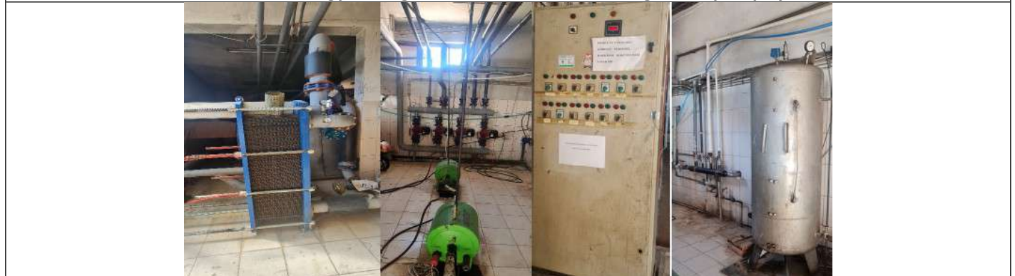
Geothermal energy management center, heat exchanger and pump systems
