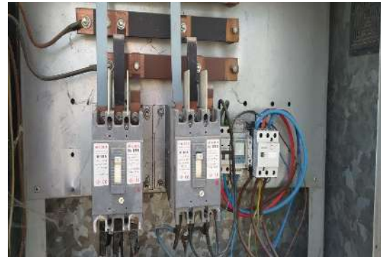
Smart Lighting Control
