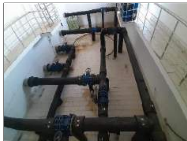
Tank distribution pumps and valves (Kütahya Dumlupınar University, Türkiye)
