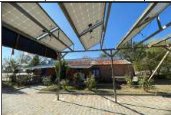
PV System Installation (180 kW)
