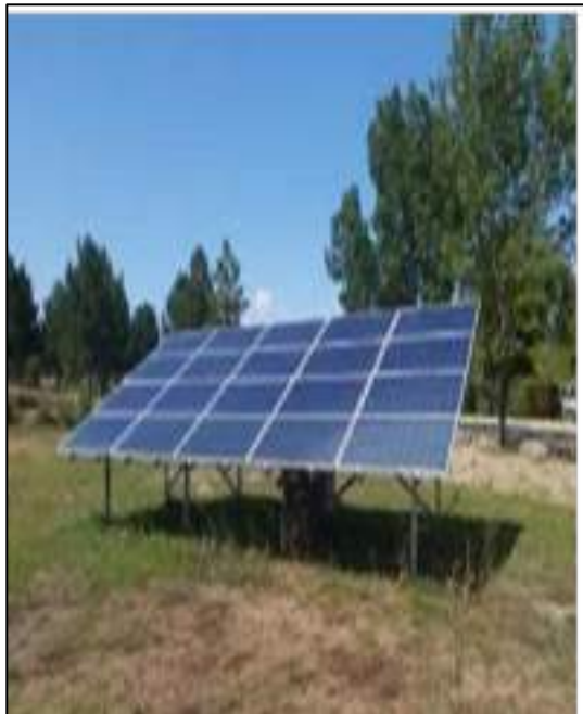
5 kWh Solar PV Energy System Connected to the Campus Electricity Grid
