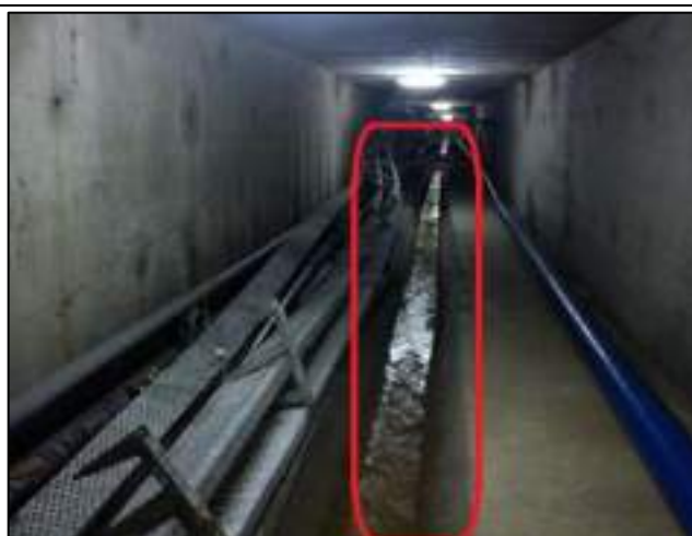
Transportation of recycled rainwater from underground to reservoirs (Kütahya Dumlupınar University, Türkiye)
