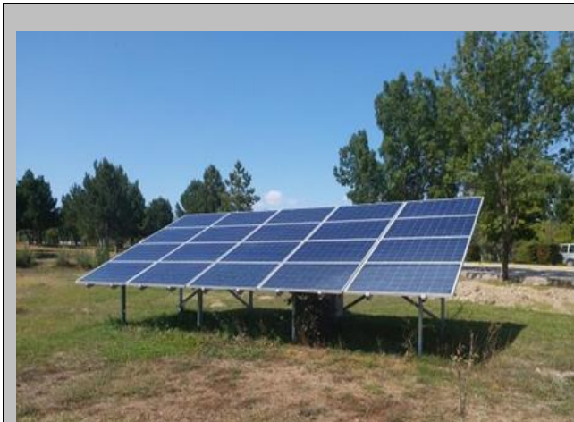
5Kwh Solar PV energy system connected to campus electrical grid. (Dumlupınar University, Turkey)
